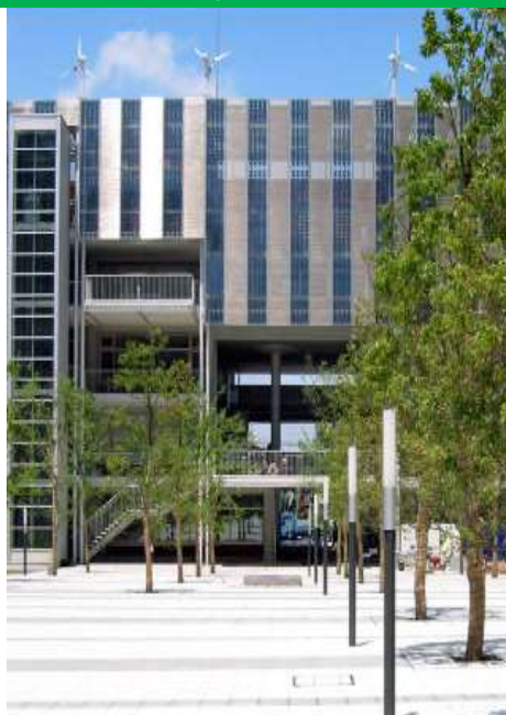
⑤ Solar Curtain Wall (BIPV) Type SKY SOLAR for the Building Facade Daito Bunka University lecture House Curtain Wall
