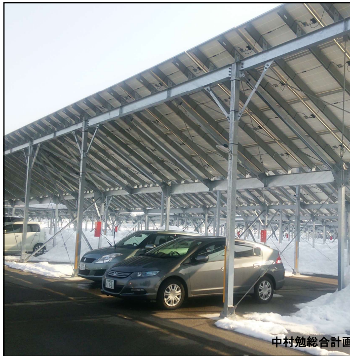
Aizu Wakamatsu Carport Type 1.3MW
